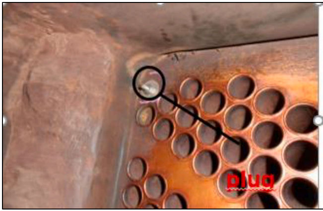
Fig. 9. Detached plug found in the condenser waterbox.
